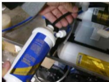
5. Connect it into outlet of sediment filter
