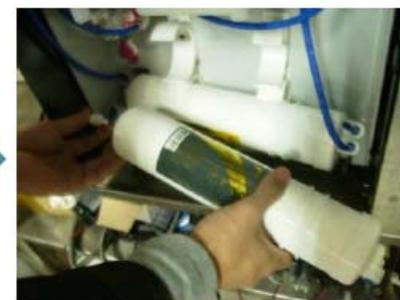
8. Connect in tube completely and put the filter in
