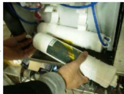
3. Prepare the tube for filter flushing
